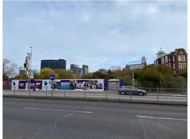
Photo 4: Looking east Anglesea Road
