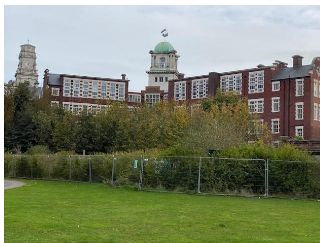
Photo 2: The site and north elevations of the Park Building, with the Guildhall tower to the left.
